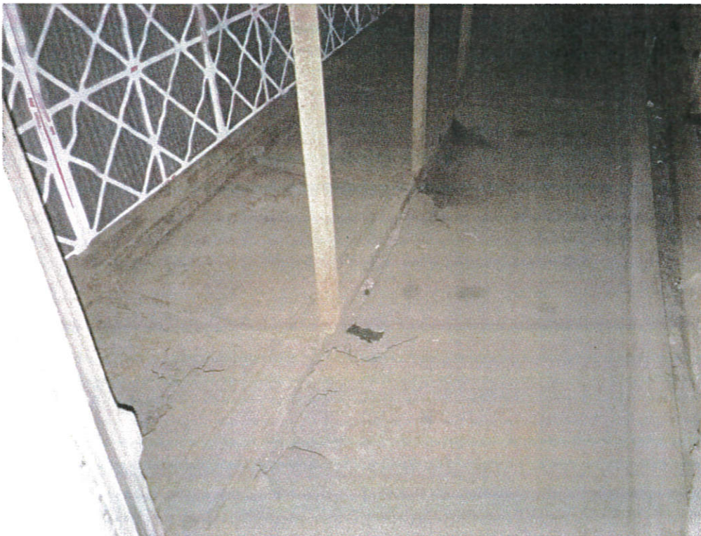
Holes in the intake ducts that result in cooling and heating loss.
