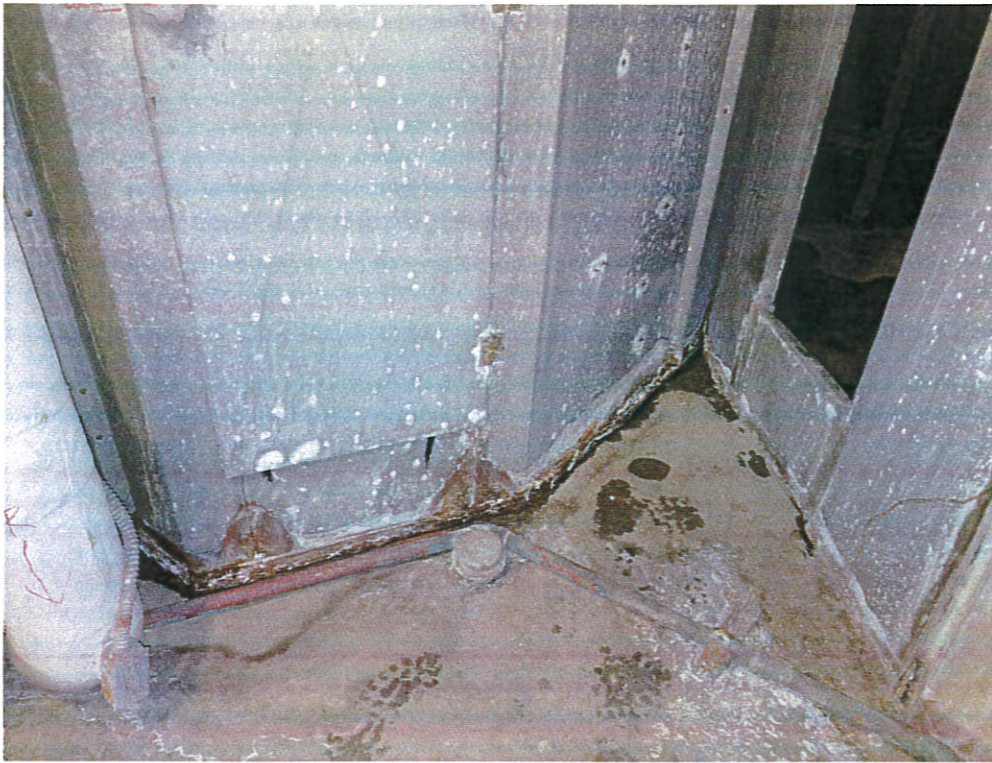
Base of air handler unit completely corroded and rusted out.
