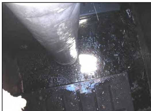
Removal of trash, sediment and debris.
