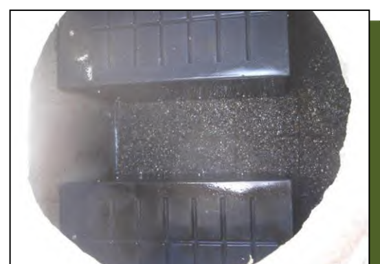
Fully cleaned separation chamber.
