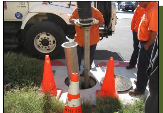
Insertion of vacuum hose into separation chamber.
