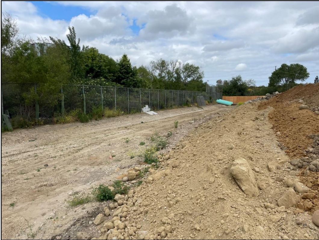
Photo 1: Facing, west. Overview.
