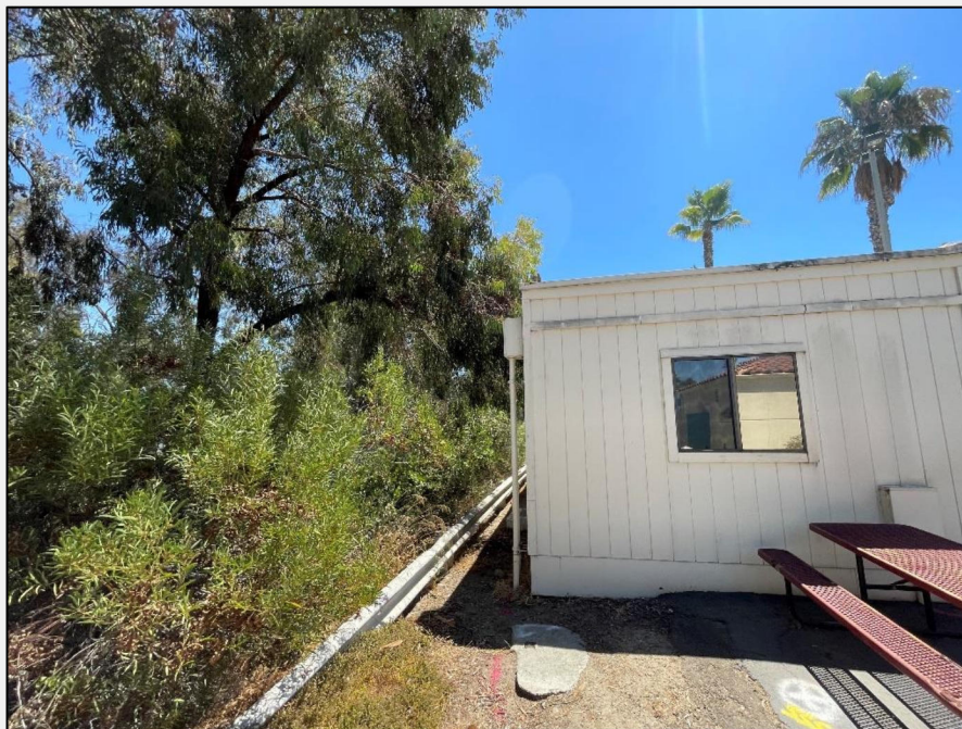
Photograph 18: Example photograph of the eucalyptus understory southeast of the Peninsula area and the proximity of the vegetation to existing structures. Photograph taken north of the SDSU Passport office looking south
