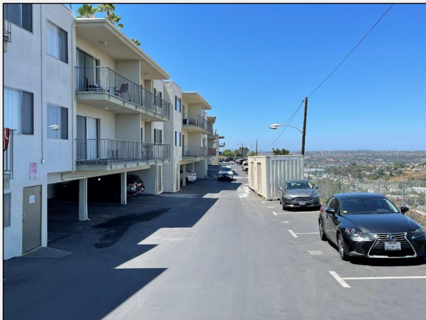
Photograph 10: Overview photograph of the existing setback of structures from the top of slope at the northern portion of the Peninsula area. Photograph taken from the northeastern corner of the area facing west.
