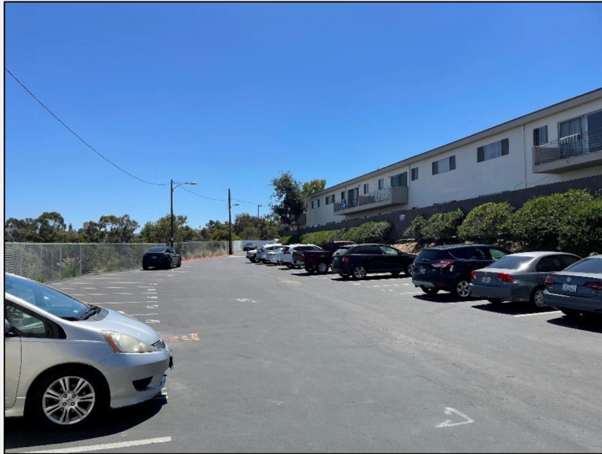
Photograph 7: Overview photograph of the existing setback of structures from the top of slope at the northeastern portion of the Peninsula area. Photograph taken from the northeastern corner of the area facing south-southeast.
