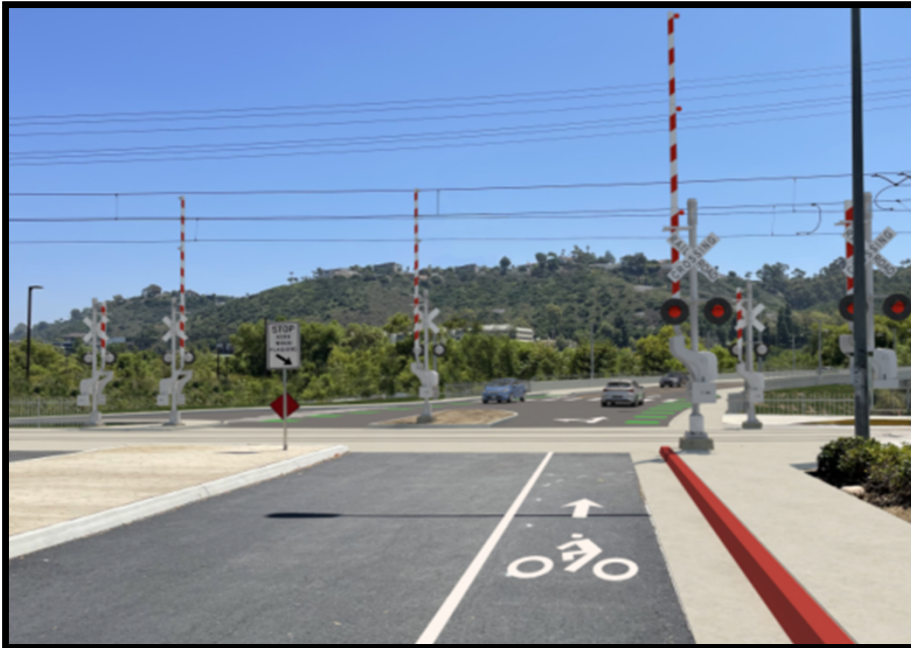
View looking south.
