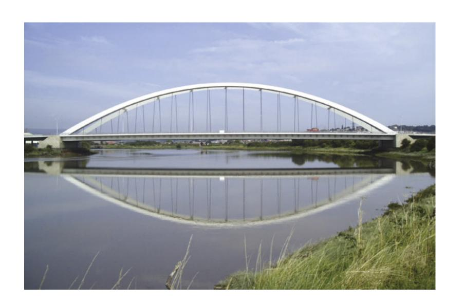
FIGURE 5-2 Tied-Arch Bridge Example Fenton Parkway Bridge Project EIR
