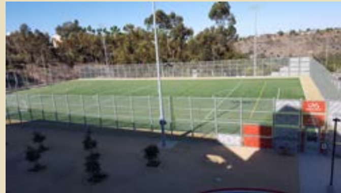
FIGURE 5 Chain link fencing appropriately used at the new student recreation field.
