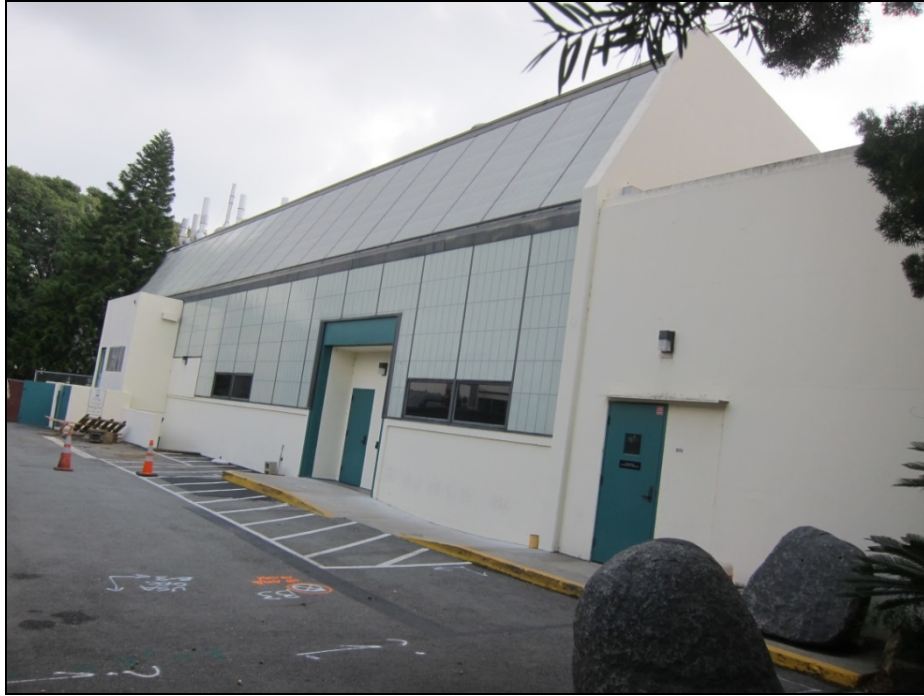
Figure 10 North Elevation of Industrial Technology Building in 2015 (view to SE)
