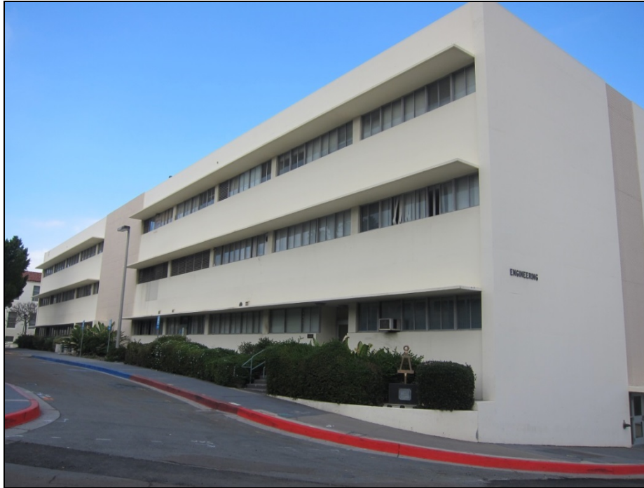
Figure 13 South Elevation of Engineering Building in 2015 (view to NW)
