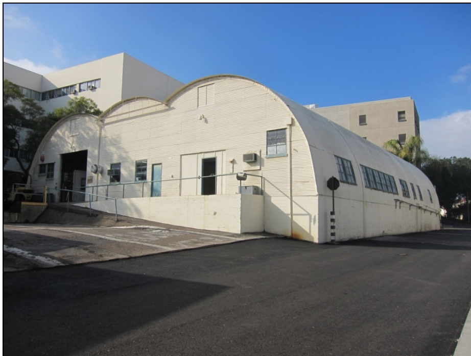
Figure 8 Facilities Services Building (view to SW)
