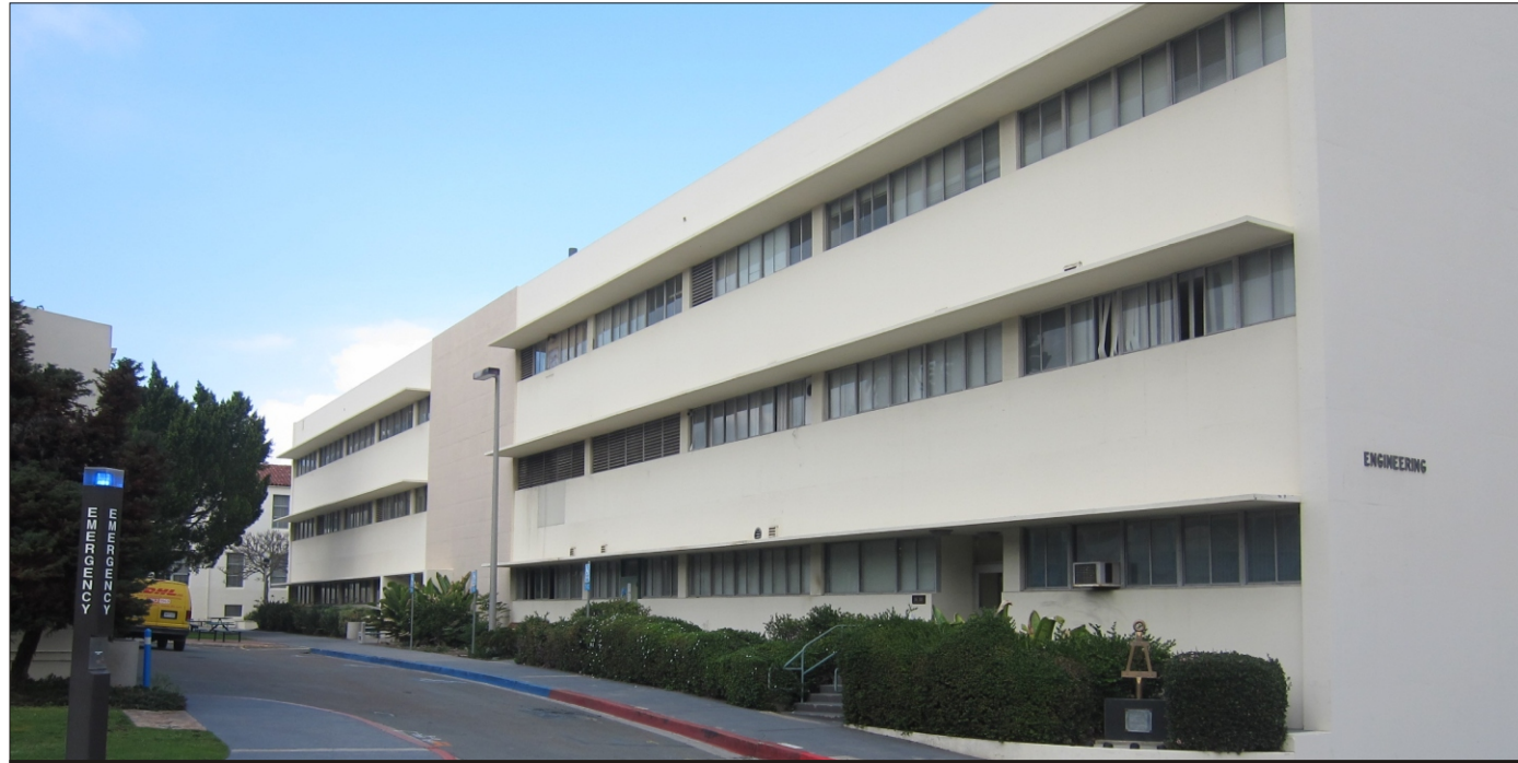
View 7 – View of Engineering Building from Aztec Circle Drive
