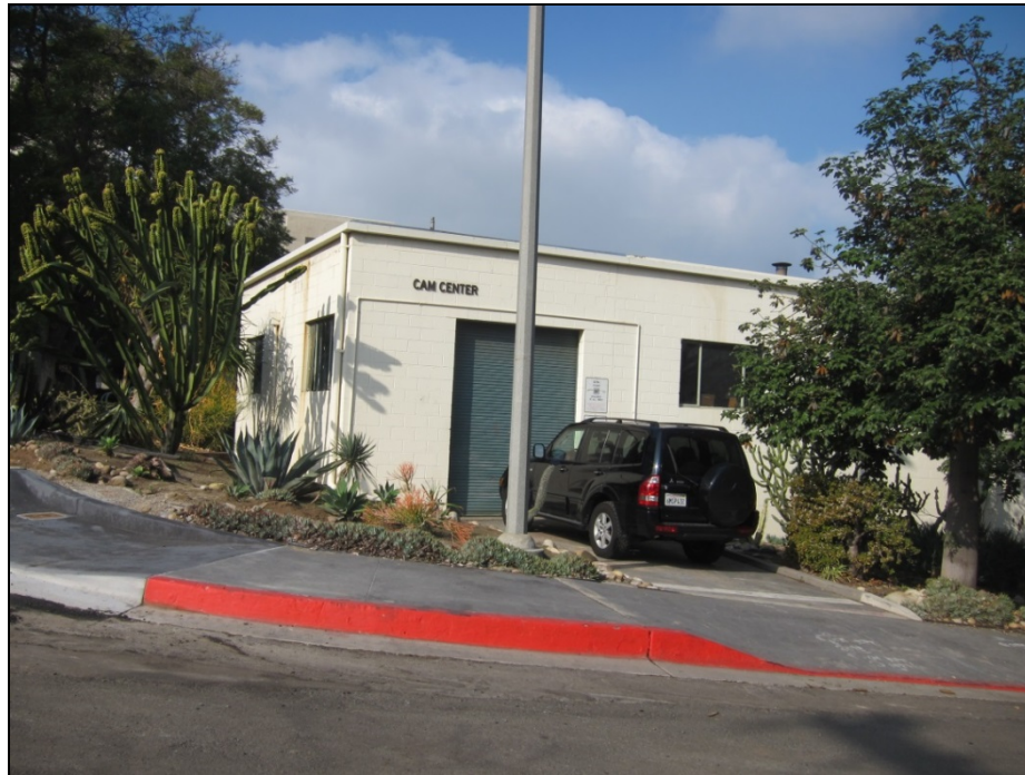
Figure 14 CAM Center (view to west)
