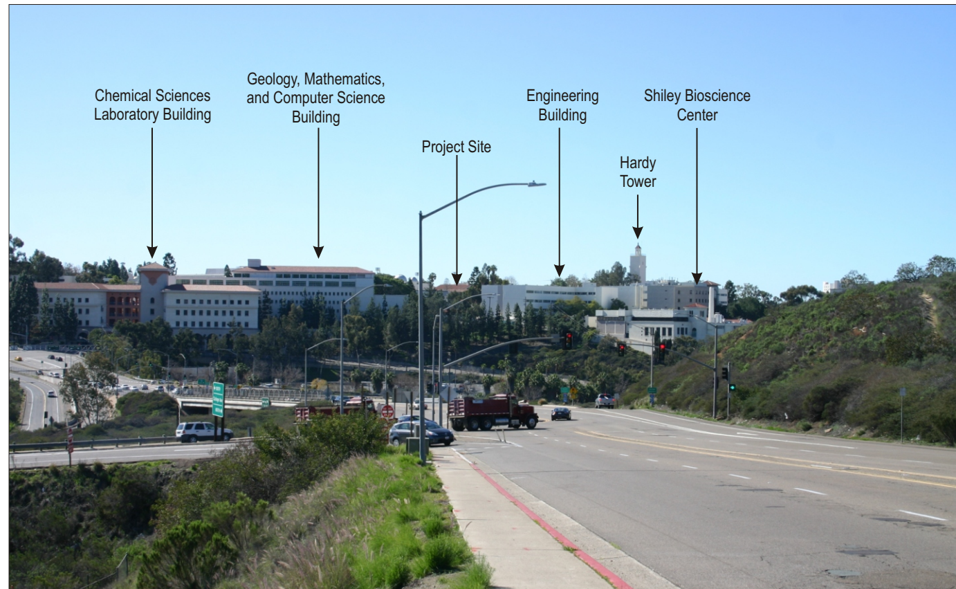
Existing View Mobile viewer traveling south along College Avenue
