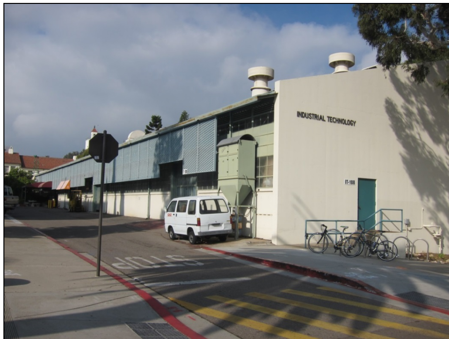
Figure 9 South Elevation of Industrial Technology Building in 2015 (view to NW)
