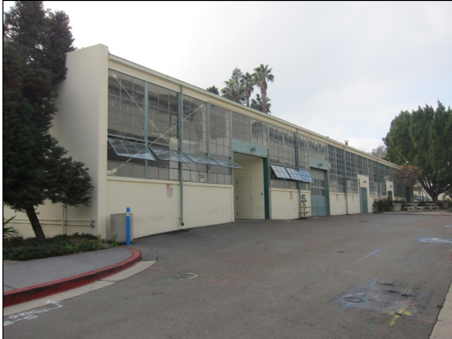
Figure 12 North Elevation of Engineering Laboratory Building in 2015 (view to SW)
